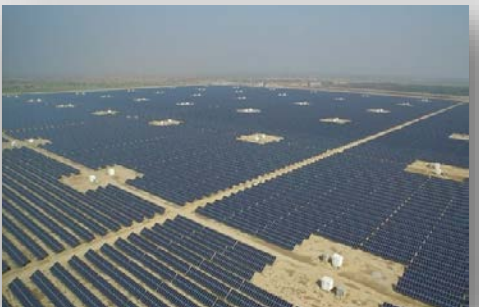
Pakistan 900MW Surface Power Station
