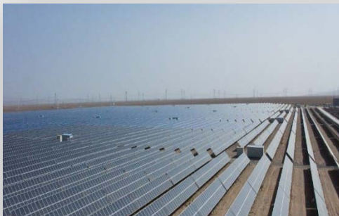
Ukraine 200MW Surface Power Station
